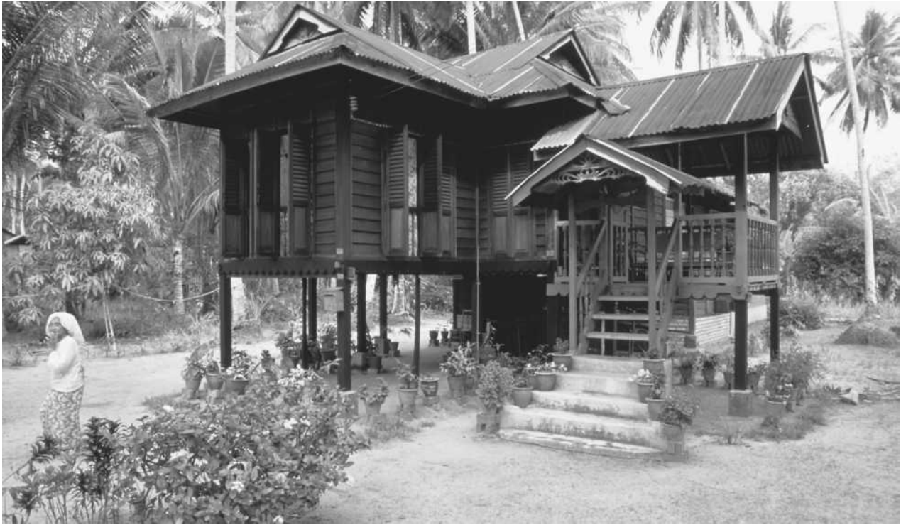
A house on Langkawi Island. Land ownership is a controversial issue in Malaysia, where indigenous groups are struggling to protect their claims from commercial interests.
